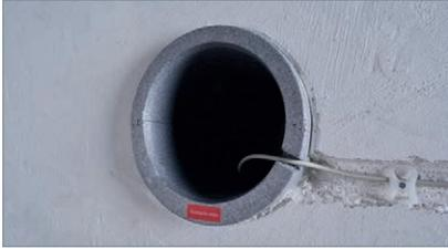
Insert the connection pipe (min.  $3 \times 0.60 \text{ mm}^2$ ) laterally (room-side view) into the wall duct. Allow the connection pipe to protrude in **length past the wall duct**.
