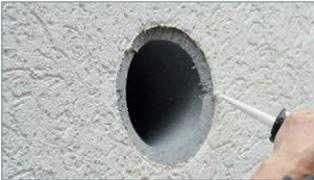
To protect against water penetration into the wall opening, the facade-side transition to the wall duct must be sealed **circumferentially** using a suitable sealant!
