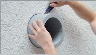
After completion of the insulation / plaster work, remove the wall covers on the interior and exterior side. Adapt the wall duct to the dimensions of the finished wall by trimming the wall duct flush with the **room** or **facade side** using a carpet knife or a hot wire.
