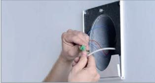
Subsequently, connect the plug connectors of the connection line to the **controller** (for details see Electrical connection **Page 10**).
