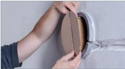
Close the wall duct on the interior and exterior side using the supplied wall covers (**see Page 14**), in order to prevent contamination of the wall duct.
