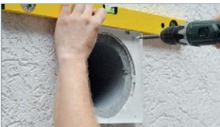
Subsequently, install the wall panel to the weather protection hood using suitable attachment elements.
