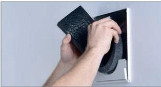
Circumferentially insert the sound insulation mats with a distance of min. 3 cm to the ventilator unit on the room side.
