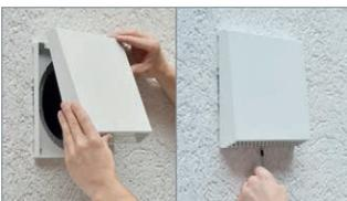
Install the weather protection hood to the **AirUnit**. The hood is mounted onto the attached brackets on the upper edge of the wall panel and attached to the wall panel using the supplied attachment screws.
