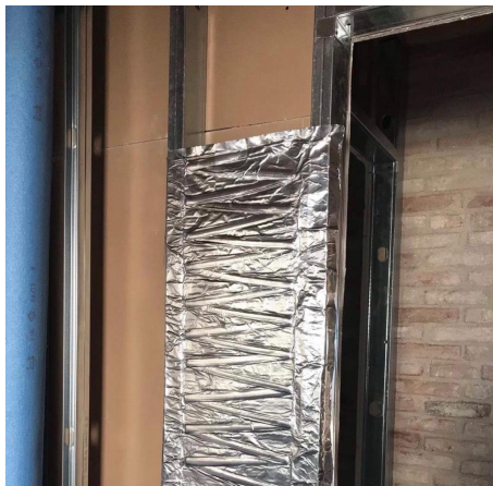
Installation Warmdrywall on drywall
